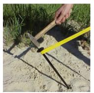
get four positions for the sand anchors to fix the net posts. At last hammer the sand anchors into the sand at a pointed angle.
